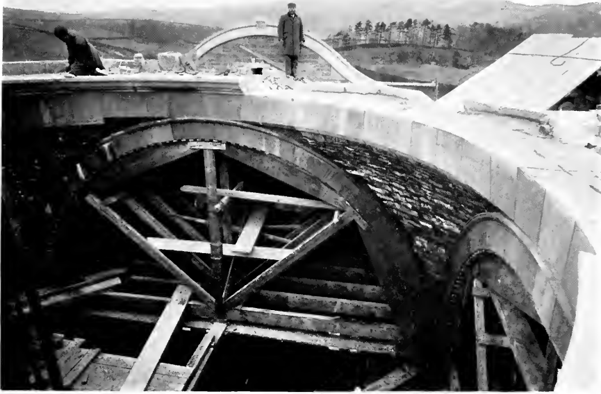
THE DOME IN CONSTRUCTION
